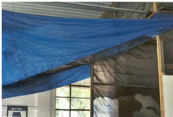
Figure 9. Spray room at Company B
